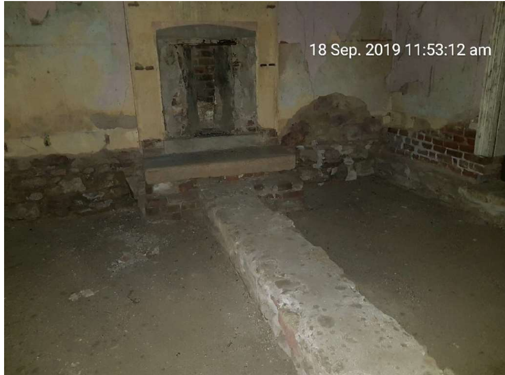
Figure 13: Inside Overdene Homestead September 2019
