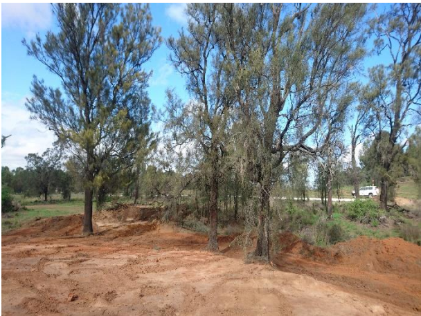
Photo 3.1 Stage 2 – clearing – GDP 1901
